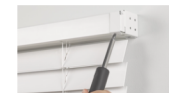
If you need to remove your blind, remove valance and use Flat Head screwdriver to pop open brackets.
